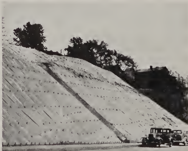
Cotton fabric of a special type prevents damage to cuts and fills in road building.
